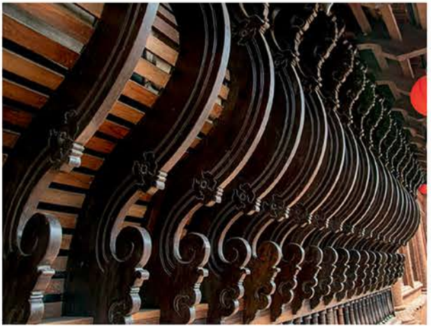
Traditional carved wooden beams on the third floor.
